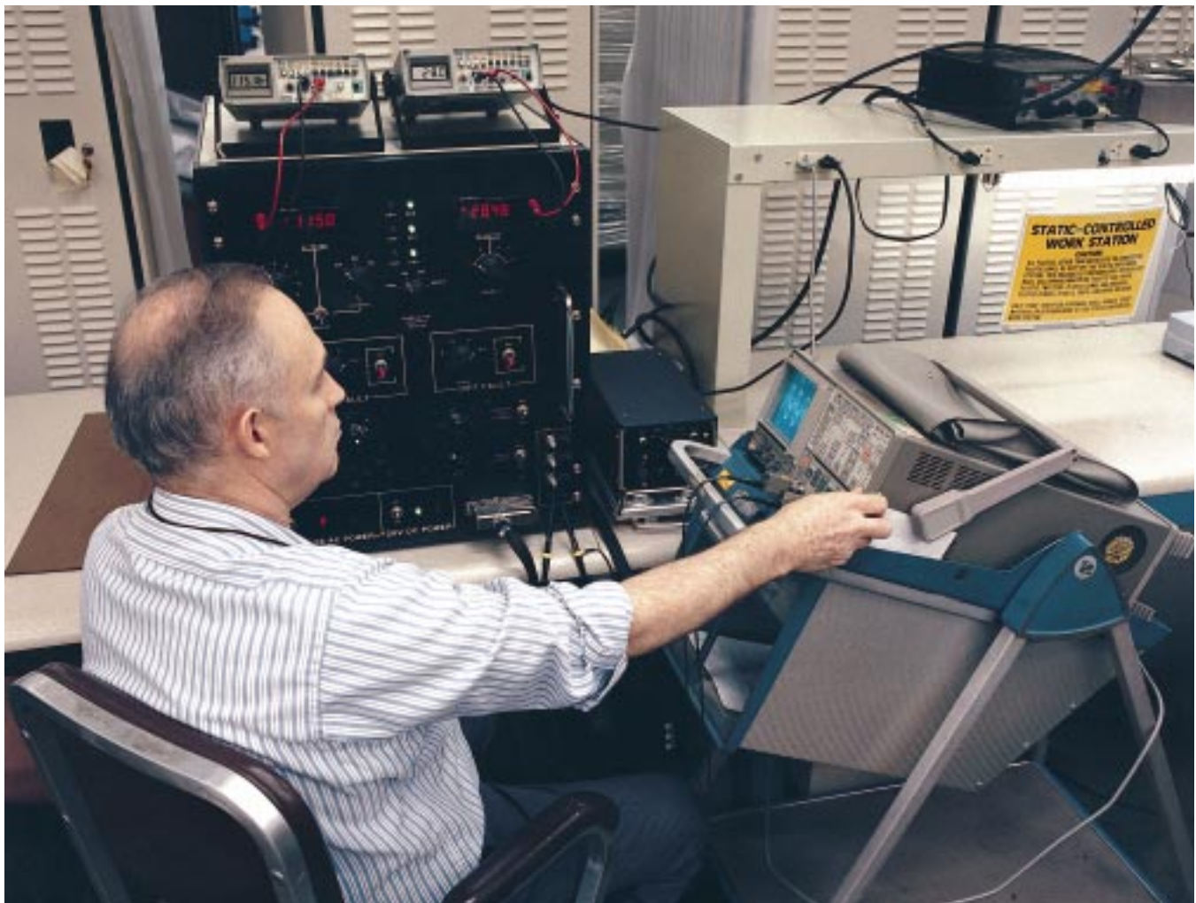
Repairing an AC generator control panel, using the PN 3402749-5 test set.
