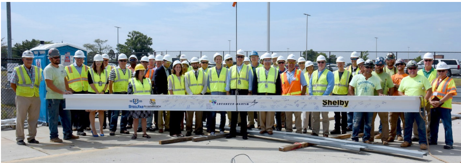
Representatives from the Lockheed Martin LRDR team and construction partner Amec Foster Wheeler stand behind their signatures on the final beam of the LRDR Integration Site.
